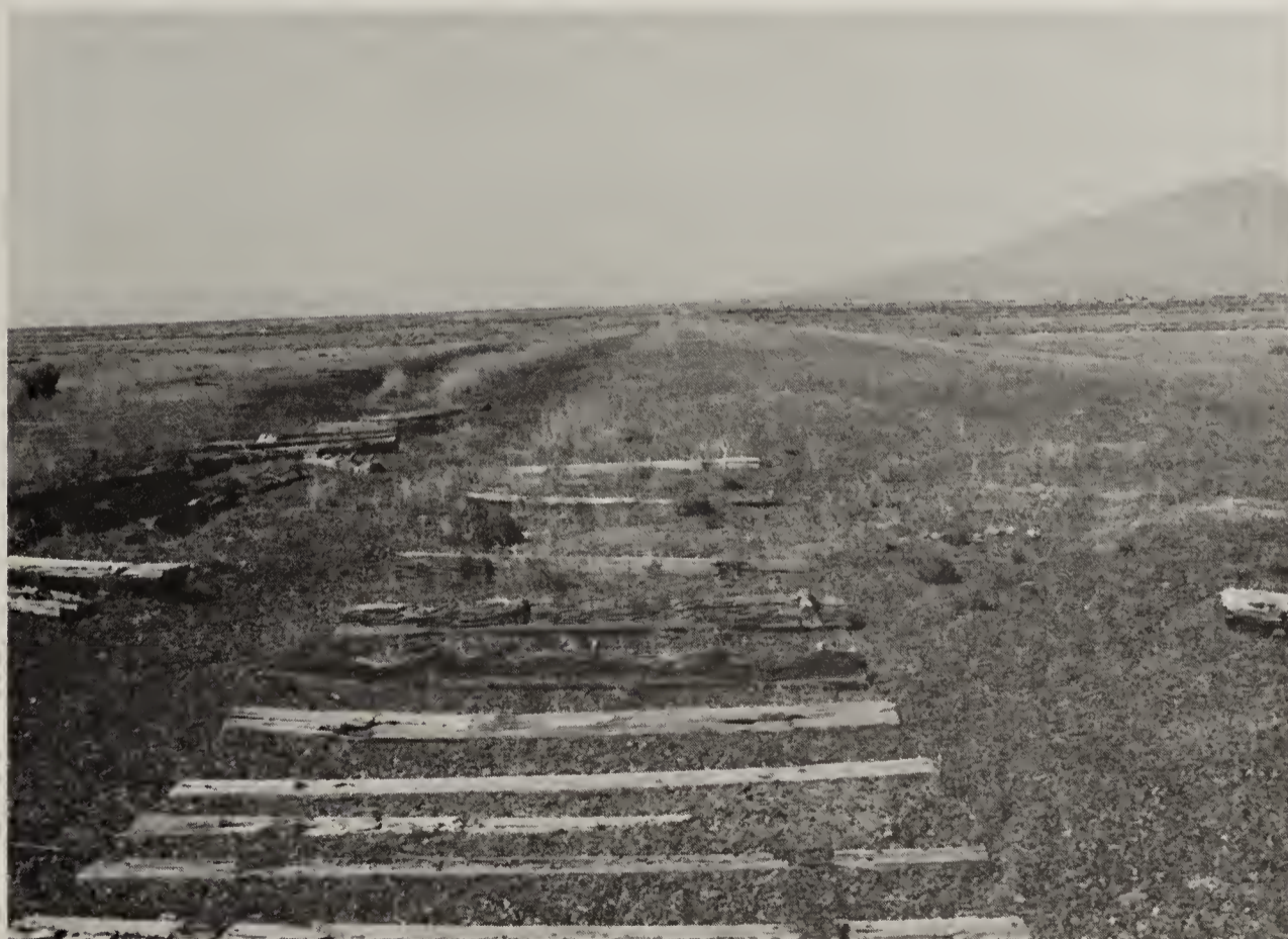
Figure 34: Terrace switchyard looking west (BLM photo)
